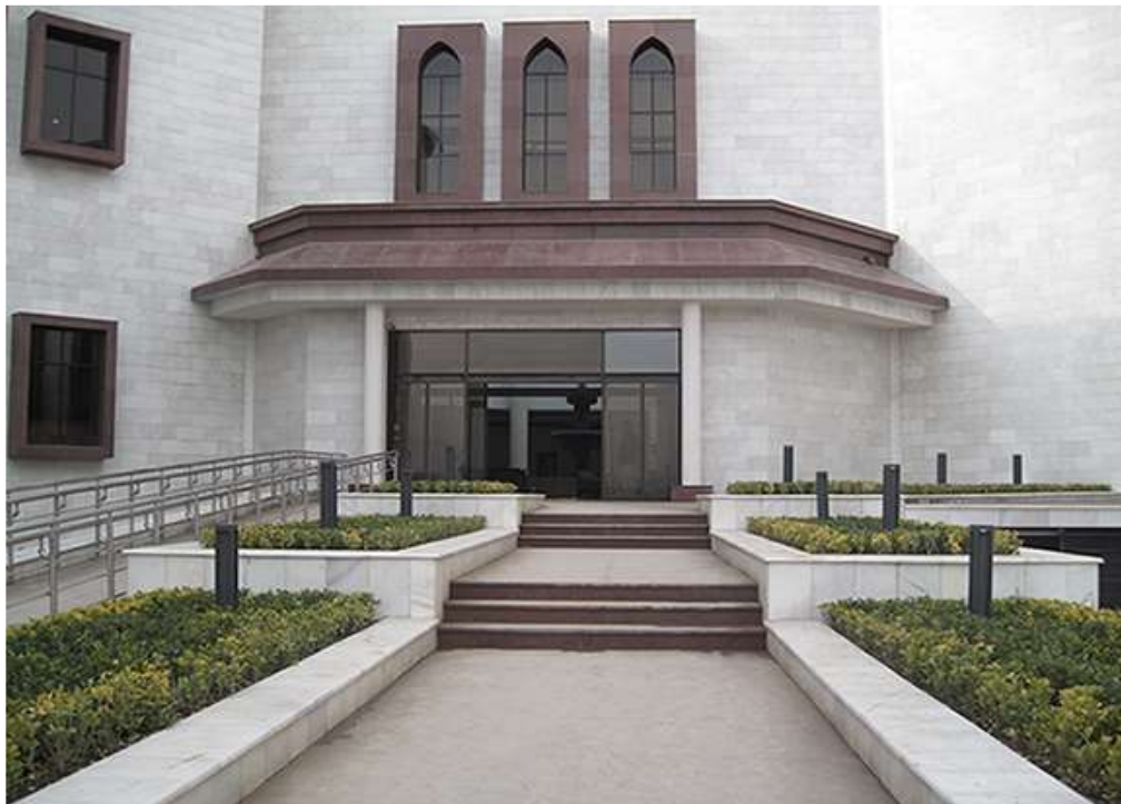
South east subsidiary entrance with a ramp for the handicapped leading to the ceremonial hall
